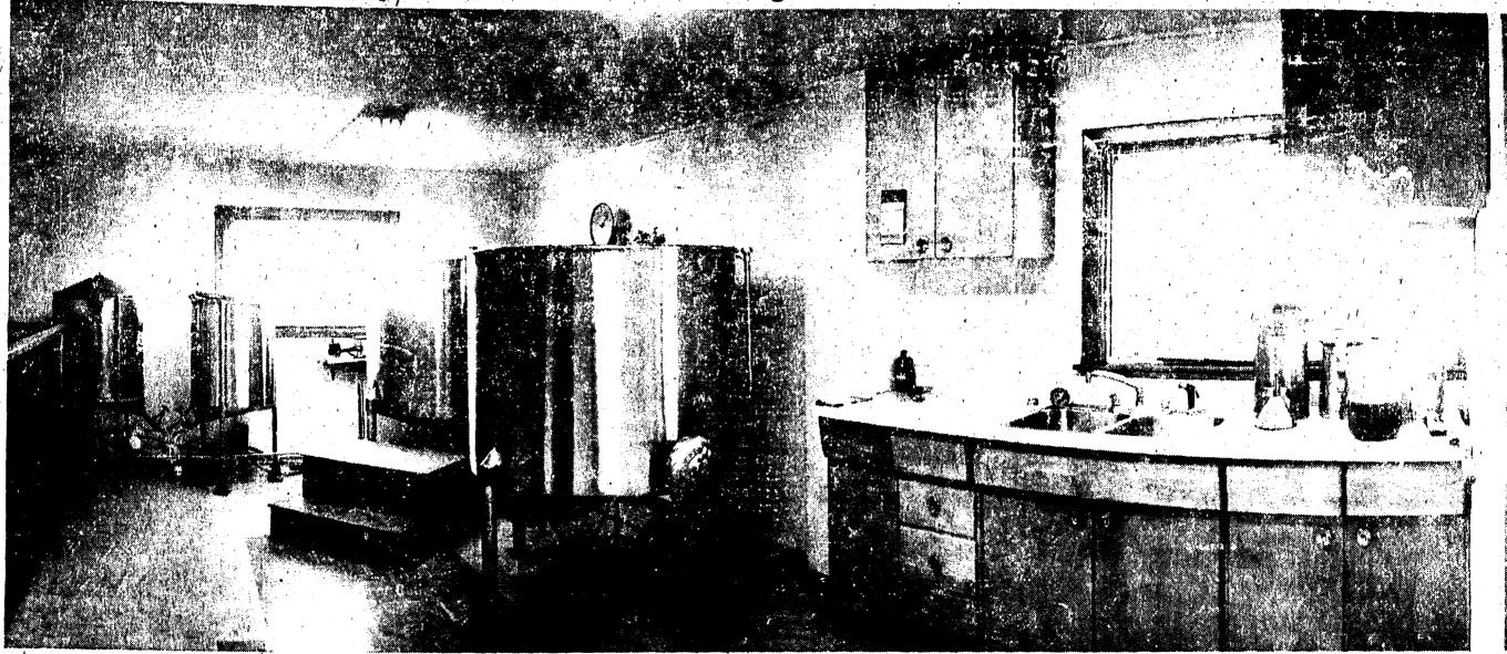
The manufacture of the bottling syrup at Jones Bottling Co. Ltd's. new Weymouth plant takes place in this room in which are installed two 300-gal, and two 50-gal, stainless steel mixing tanks connected by stainless steel tubing.
