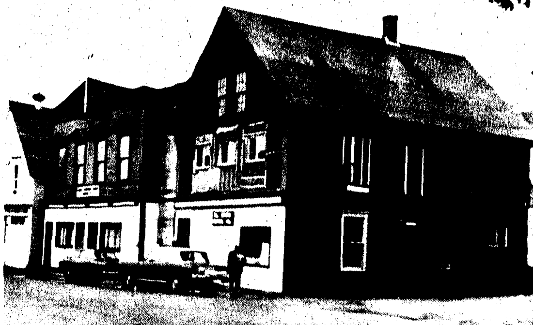
Two buildings in the business section of Bear River which are owned by the Bear River branch of the Canadian Legion have been joined together. The second floor covers the entire space of the two buildings together. The walls separating the two buildings were removed and thus making one large room. On the ground floor, the middle building shown in the photo, will serve the local ladies of the branch and the ground floor of the first building to the left, will serve as a drop-in and activity centre for the Bear River New Horizons, which they are presently occupying. The Legion branch allows the New Horizons club use that portion of the building rent-free, a generous gesture on the Legion branch's part. (Melanson Photo)
