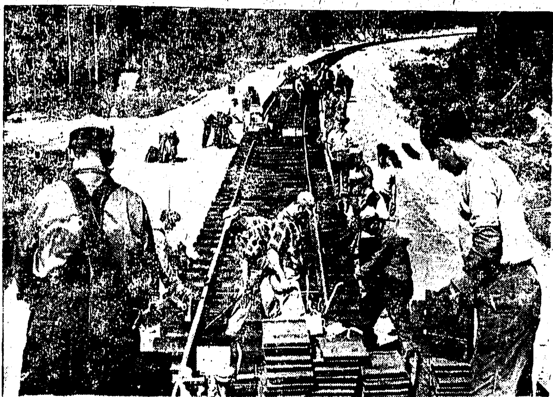
SPIKING — Modern equipment may have displaced the sledgehammer, but building a railroad is still hard work. Canadian National Railways is using 100 men to construct a 15-mile spur from Nipisicuit Junction near Bathurst to the site of Brunswick Mining and Smelting's concentrator in northern New Brunswick. The operation pictured here is known as "spiking". Men on the end of a slowly moving flat car pass tie plates to work crews, who insert them between rail and tie. Another crew, coming along behind with an automatic driver, "spikes" rail, tie plate and tie together. The line will help develop the mineral deposits of the area. (CN Photo)
